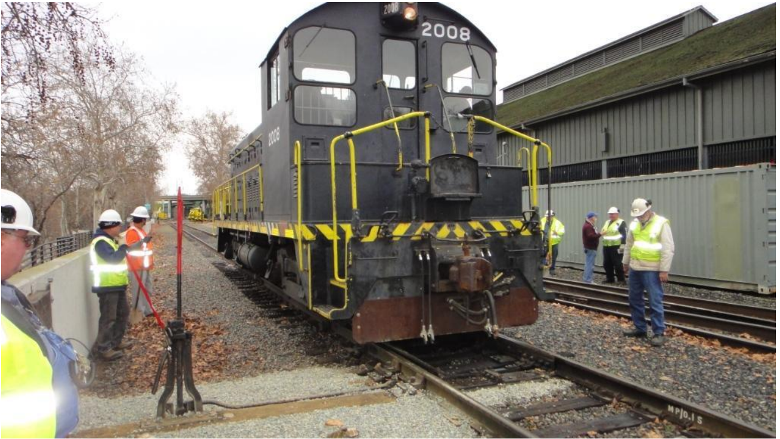
To help settle the raised switch, the SSRR 2008 rolls over it several times
