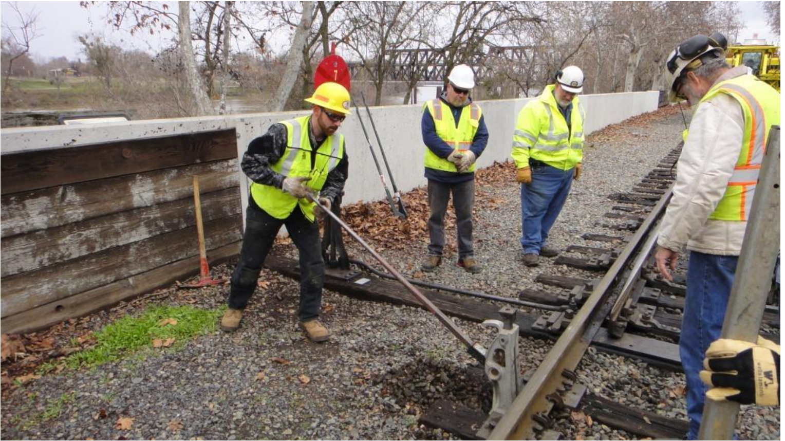
A cross-level measurement showed that the west rail was \frac{3}{4} of an inch below the east. Chris M. jacks-up the west rail
