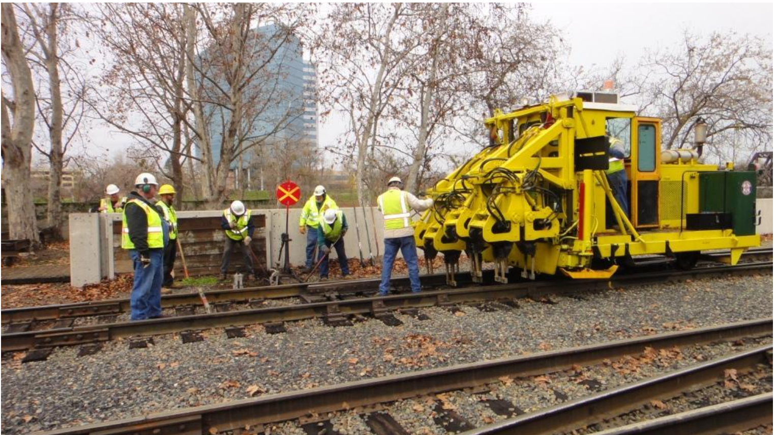
Bring in the tamper! Steve N. operates the tamper as Alan provides guidance from the ground
