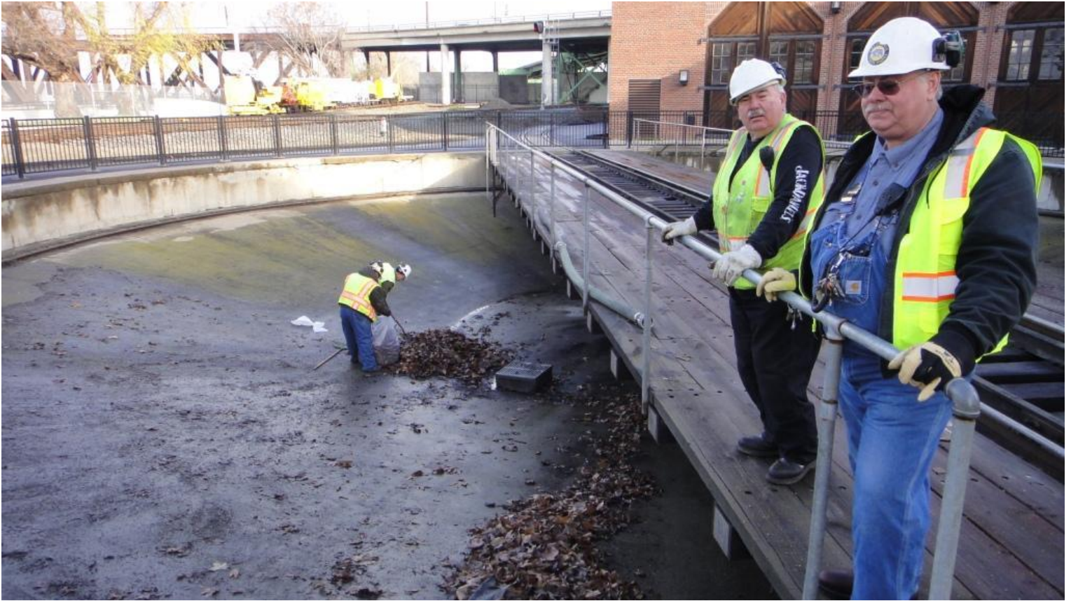
Harry and Chris C. survey the progress while Mike F. and Clem clear debris from the west side of the pit
