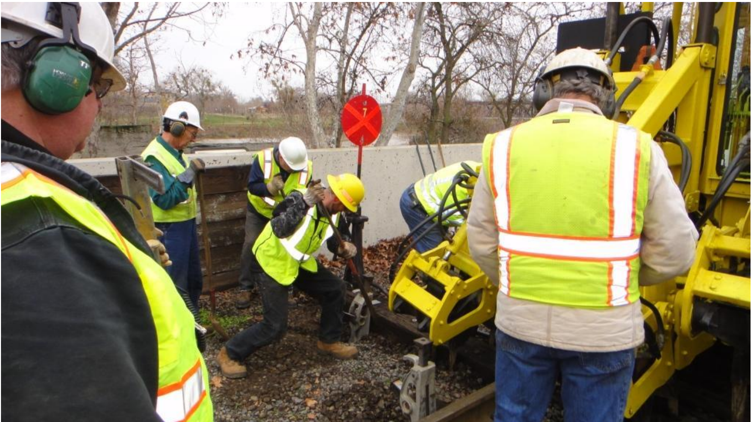
The crew continues hand-tamping the head-block where the tamper's work-head can't reach
