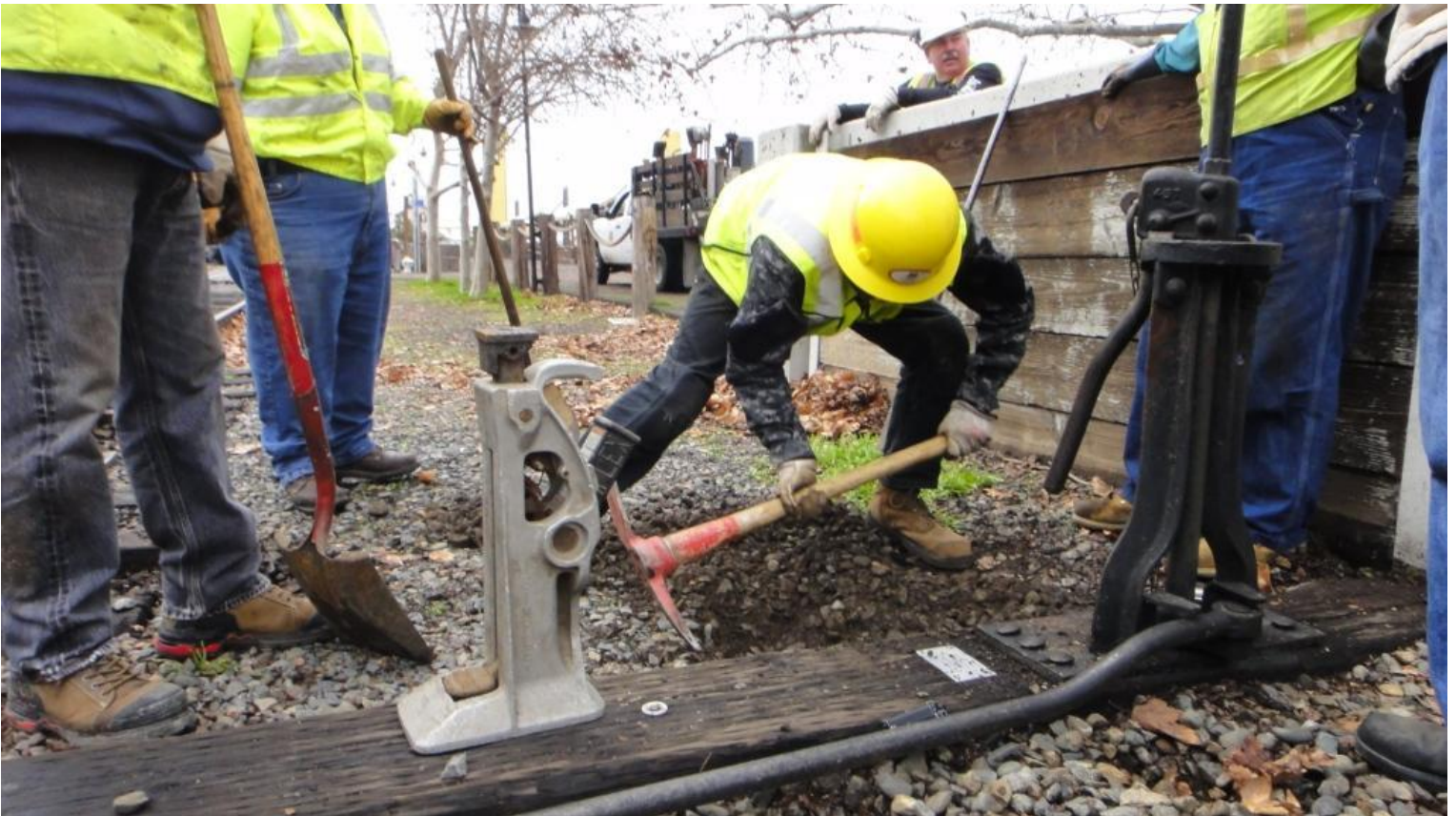
Now Chris M. digs out a space for a jack to be placed to jack-up the head-block
