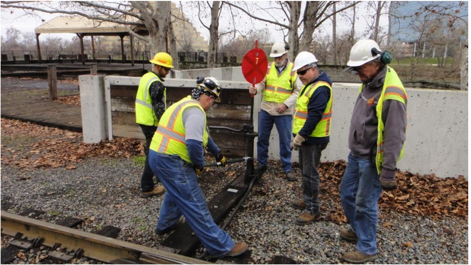
On to the next project. Mike F. uses the "Carlson Tool" to make adjustments to the stand at Switch 7
