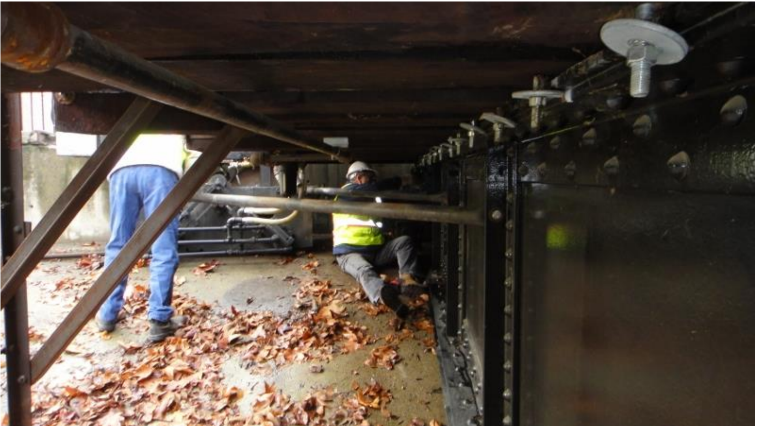
Steve W. tightens down the deck-bolts under the turntable
