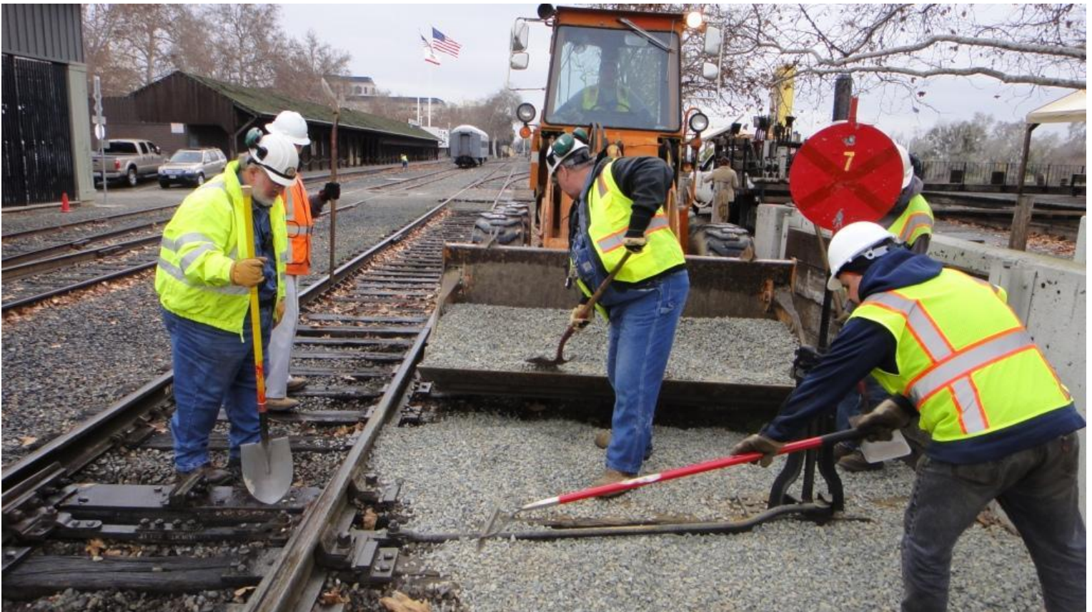
Back at Switch 7, Frank, Jose, Chris C., Steve N. and Steve W. fill in all the holes with fine rock brought over by Mike F. in the front-end loader
