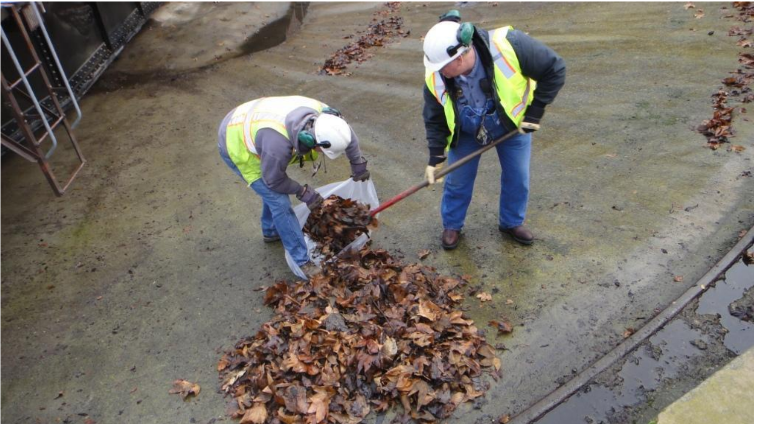
Steve N. and Chris C., clean up the turntable pit for the SSRR Crew Photo
