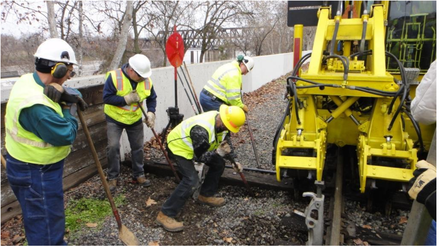
Steve W., Chris M. and Frank hand-tamp the head-block as Steve N. in the tamper tamps around the switch components
