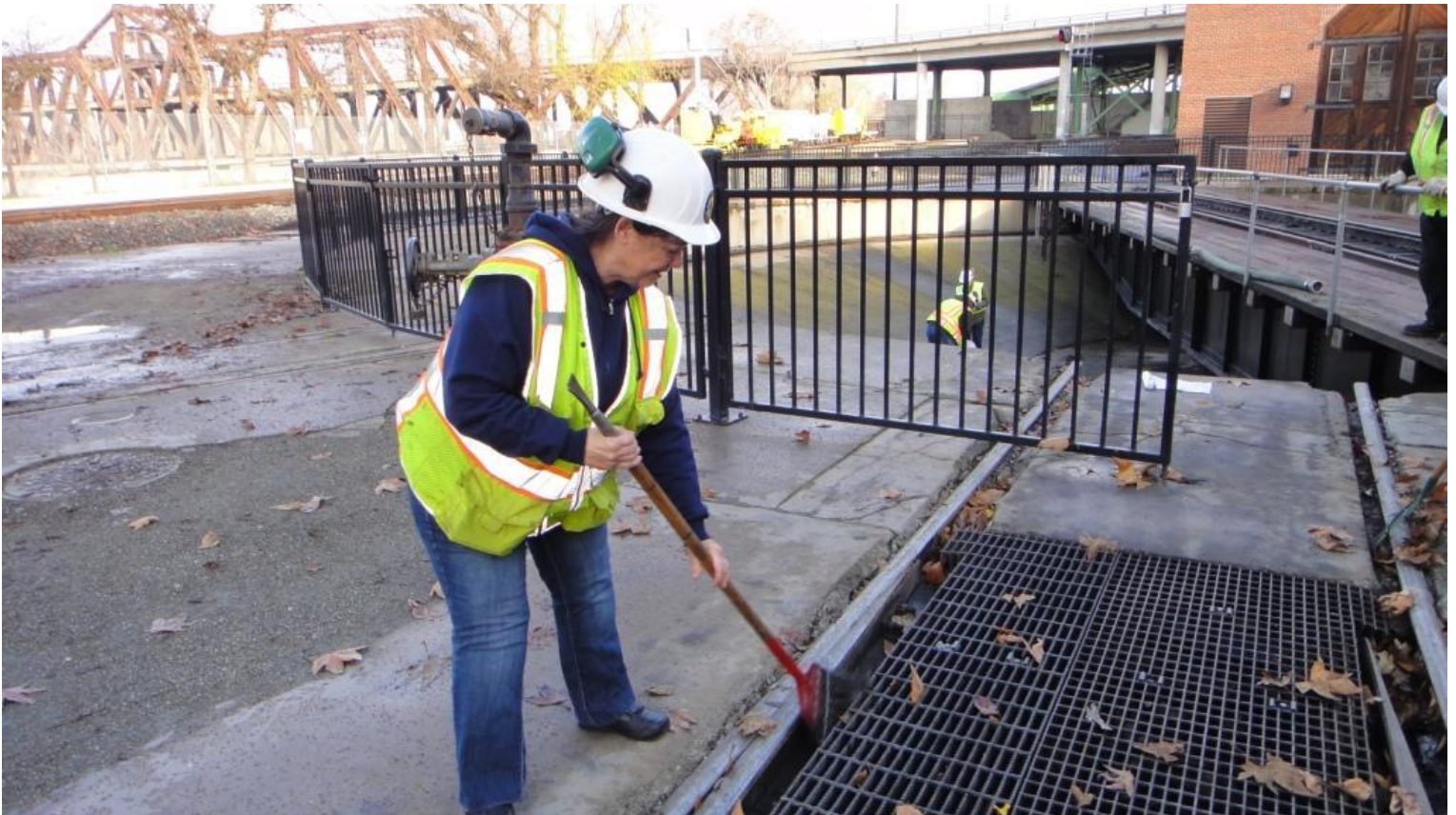
Pam clears leaf debris from the points at Switch 1
